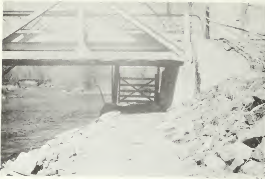
North Entrance at Boulder River Bridge
